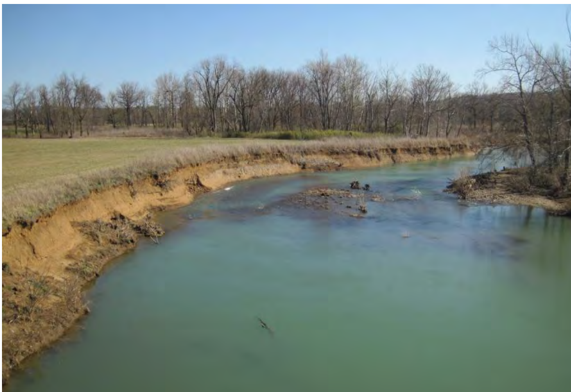
Photo 8 Area 2 looking east from Dead Horse Mountain Rd. at eroding riverbank. The 14 ft. high cut-bank will be stabilized using a toe wood bench. A riparian forest will be established on the floodplain adjacent to the restored river bank
