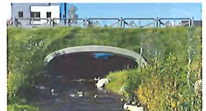
EXAMPLE OF STRUCTURAL PLATE BOX CULVERT
