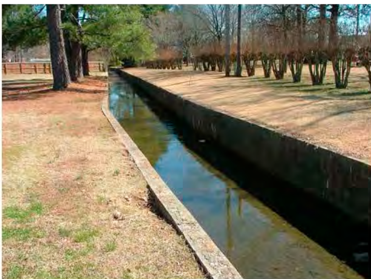
Unnamed tributary to Little Creek facing west (west of I-40)
