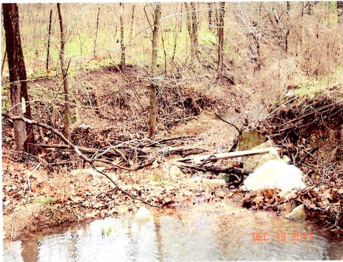
Scour Hole and Channel Incision Immediately Below the Uppermost Road Crossing on the Property
