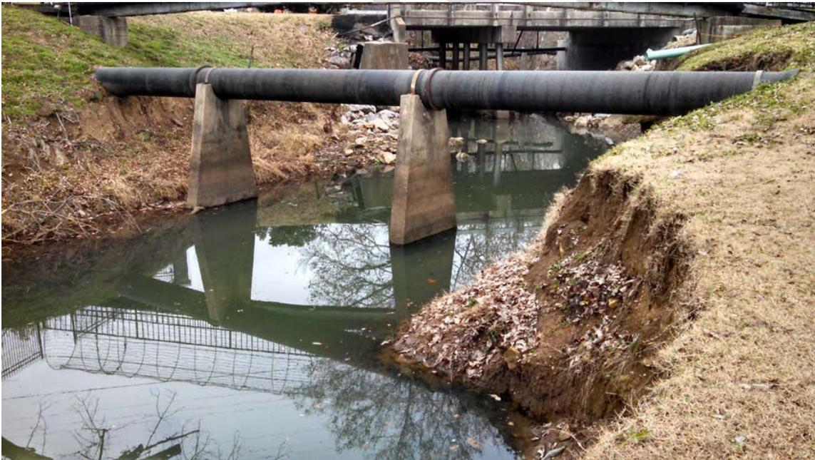
*Photograph 3: Sewer line owned by the City to be abandoned and removed prior to Construction*
