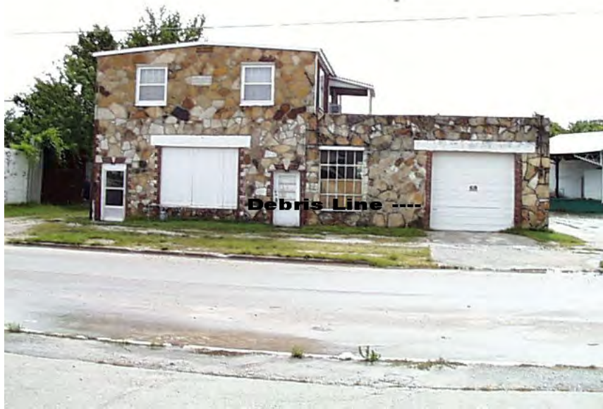
Lower Branch of Jordan Creek. 210 N Nettleton Avenue (Lower Branch RS 9211). The debris line on the garage door measures 34-inches from the floor. The FFE of the building is 1248.14, giving a WSE of 1250.97. This photo was taken after flood waters receded on July 12, 2000. See Appendix F for WSE comparison.
