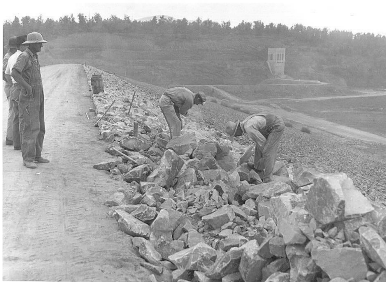
Little Rock Engineer District Blue Mountain Dam Site, Petit Jean River View looking south showing riprap being placed on main dam. July 13, 1946, 3:10 p.m. Booneville, Arkansas File B.M. 976
