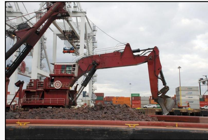
Removal of sediment and debris from the channel to allow ships to pass and maintain river flow.
