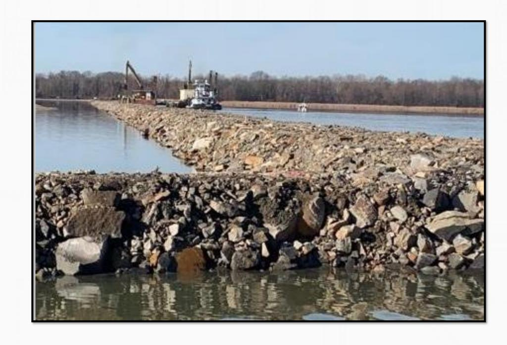
Re-directive or resistive structures that use the river's energy to deepen and enhance the navigation channel, increase environmental diversity, and maintain system status.
