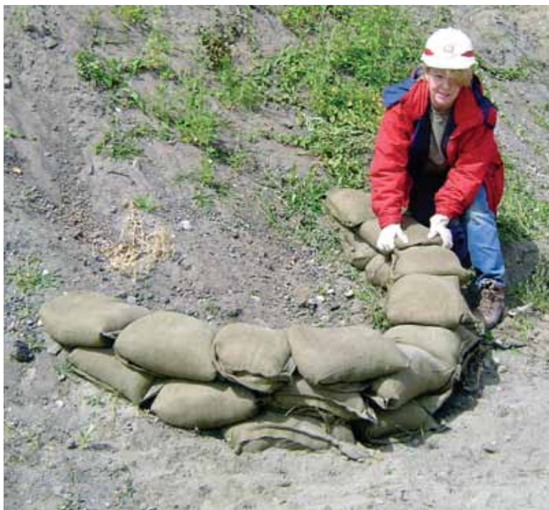
A Corps employee demonstrates building a ring dike.
