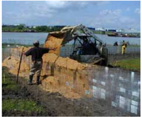
Rapid Deployment Floodwall
