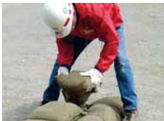
Heavy gloves provide protection from treated burlap bags
