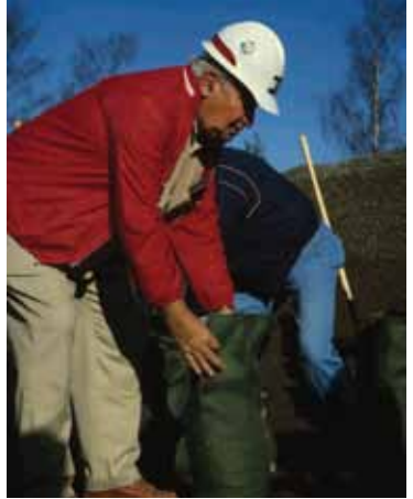
Sandbags should be two-thirds full, folded at the top.
