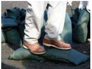
Place each succeeding bag tightly against and partially overlapping the previous one. Compact and shape each bag by walking on it.
