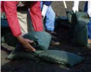
Place each succeeding bag tightly against and partially overlapping the previous one. Compact and shape each bag by walking on it.
