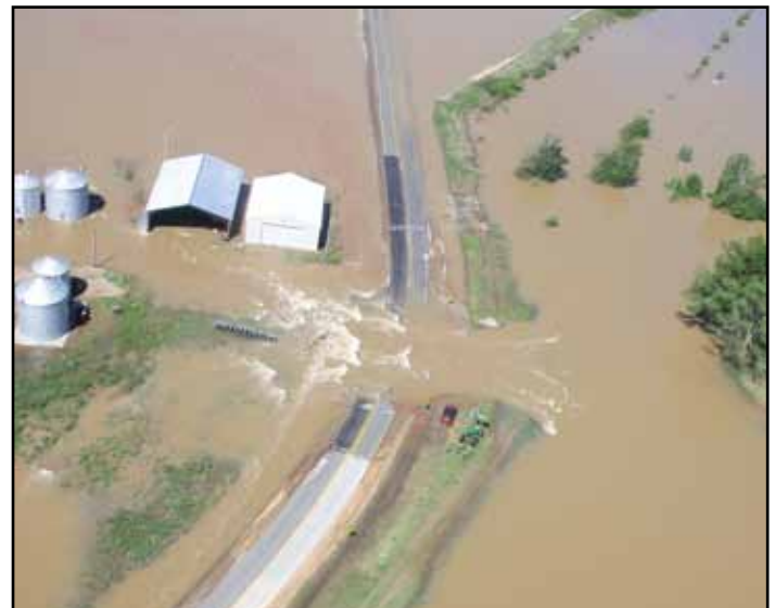
Running Water Drainage District levee breach
