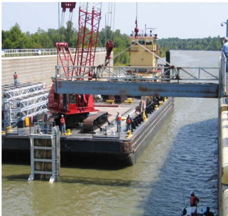
Crane barge sets stoplogs
