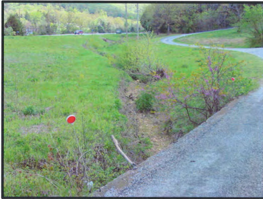
FIGURE E: INTERMITTENT STREAM CHANNEL WITHIN RIGHT-OF-WAY ON SOUTH SIDE OF HIGHWAY
