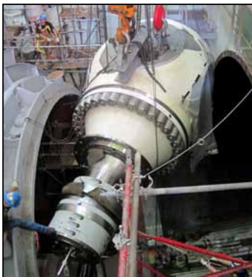
New runner being installed in Unit #2
