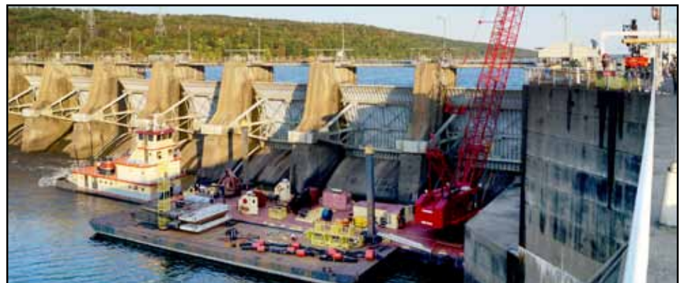
Corps personnel perform maintenance on the Dardanelle Lock and Dam.
