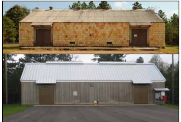
Before and after look at a Pine Bluff Arsenal's warehouse upgrade project.
