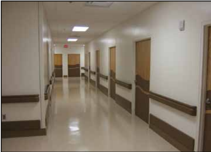
Remodeling at Audie L. Murphy Memorial Veterans Hospital, San Antonio, Texas.
