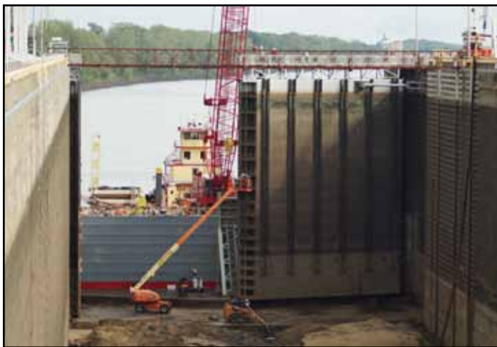
Corps personnel perform maintenance on the lock gates of Dardanelle Lock.
