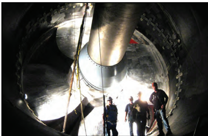
Ongoing turbine replacement at Ozark Powerhouse.
