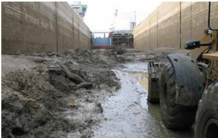
Personnel removes silt from the bottom of Montgomery.
