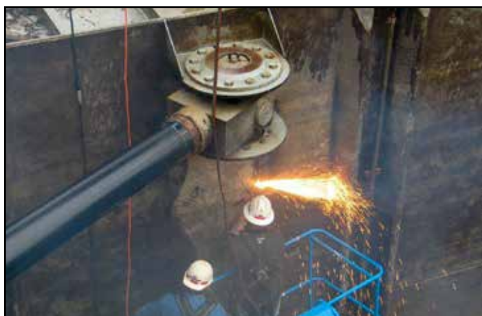
Montgomery Point hinge pin repair.
