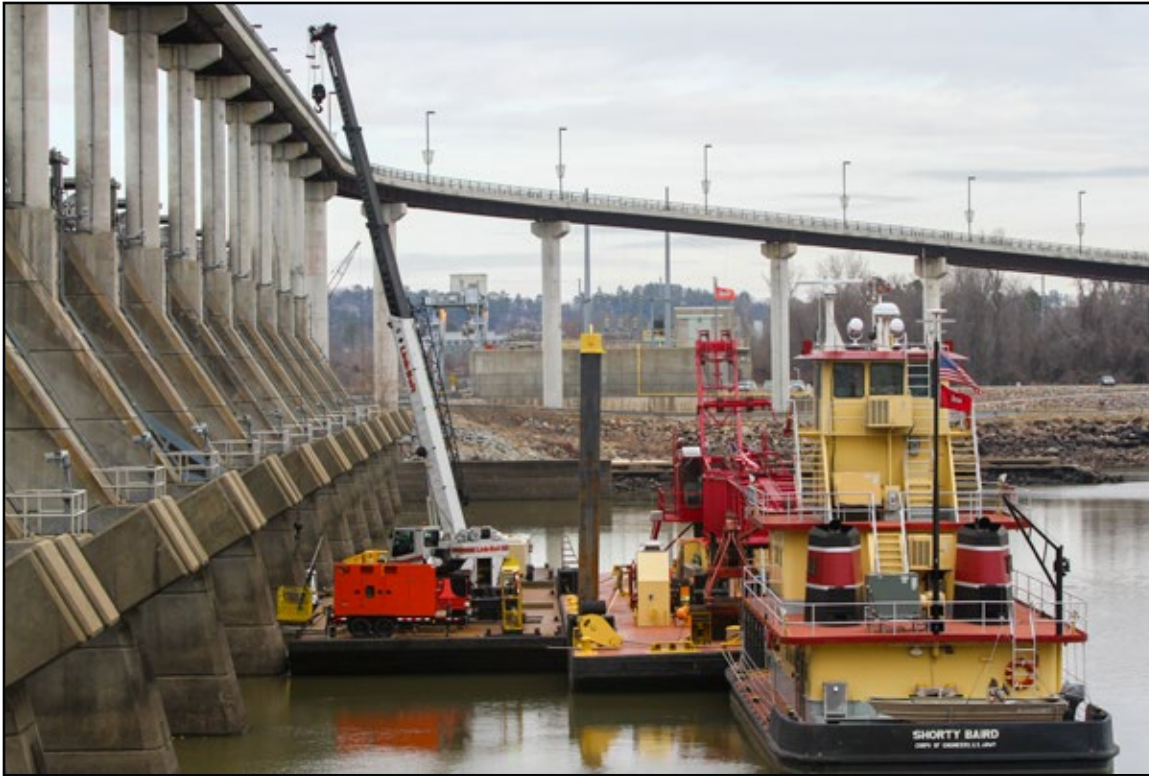
Corps personnel perform maintenance on Murray Lock and Dam
