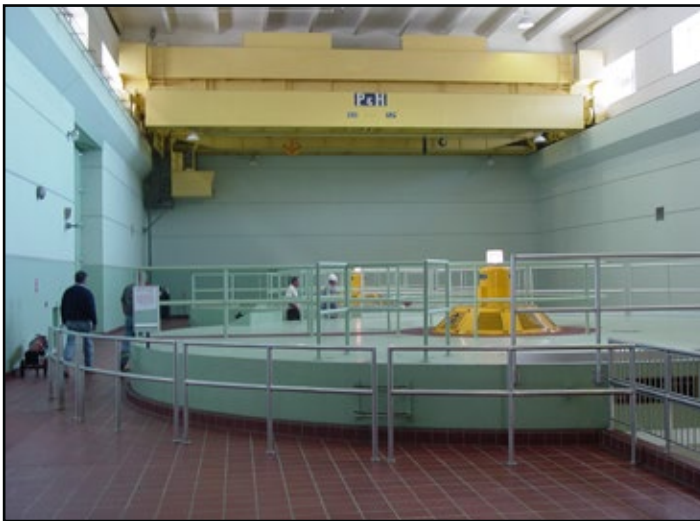
Hydroelectric generators at Greers Ferry Dam
