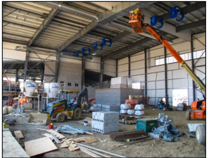
Construction work at the Little Rock Air Force Base Fuels Maintenance Hangar Facility
