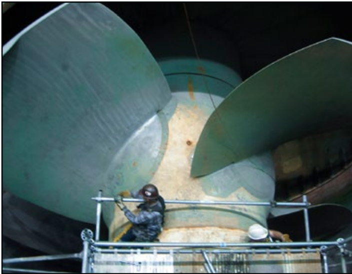
Preparing the new turbine runner assembly.
