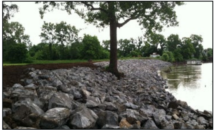
Completed Section 14, Emergency Streambank and Shore Protection Project on the White River in Augusta, Ark.
