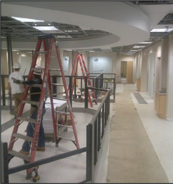
Langley Air Force Hospital renovation
